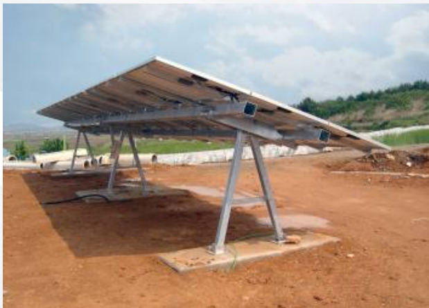
Fixed PV ground mounting
